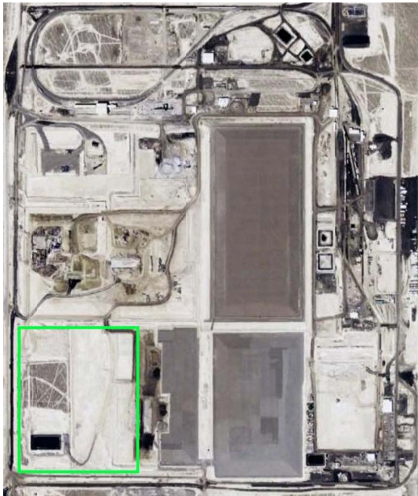
Figure 1. The Clive Facility, with the location of the Class A South embankment outlined in green. This orthophotograph is roughly 1 mile across, and north is up.
